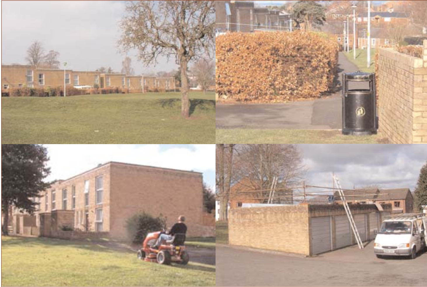
SMART work in Carlisle (Clockwise from top left) the recreation field close to the TMO office, new bin installed in 'Keep St.Martins Tidy' campaign, SMART TMO caretaker cutting the communal grassed area, re-roofing the garages - working in partnership with CHA.
